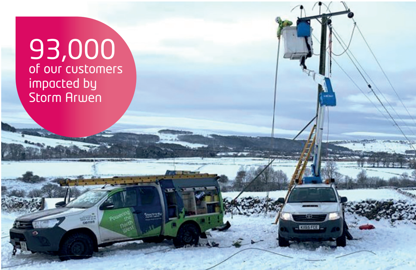
ENWL engineers repairing a damaged overhead cable during Storm Arwen
